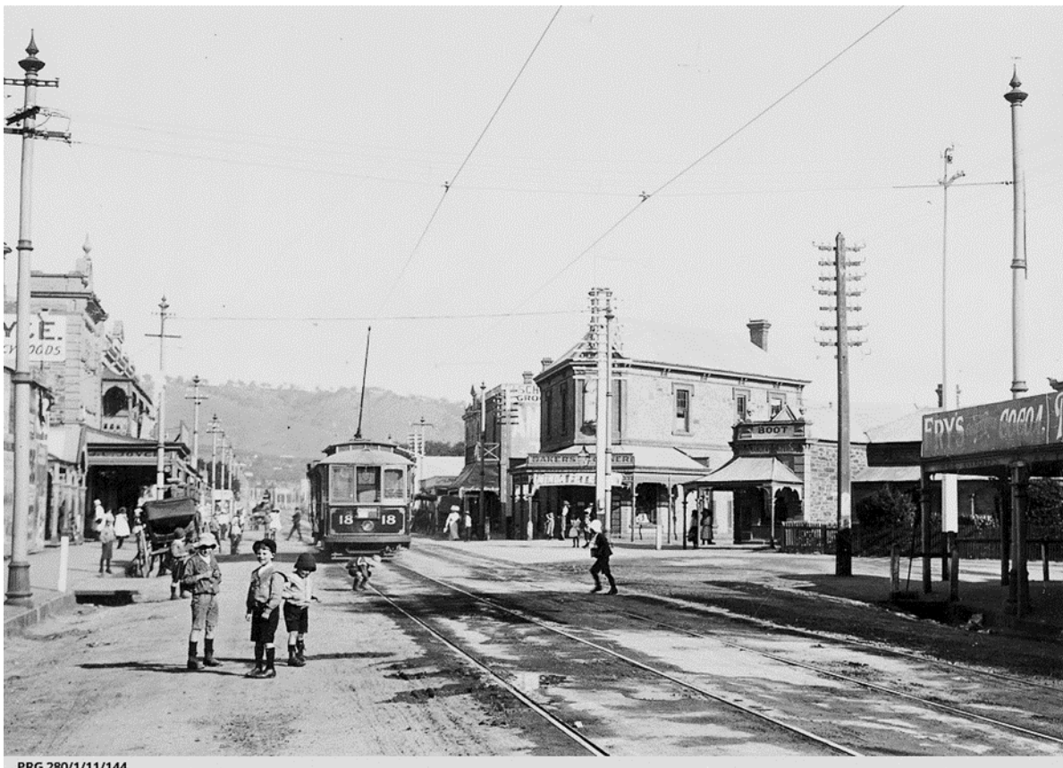
Glen Osmond Road with Kenilworth Road and Young Street on the right. 1911 (SLSA, PRG 280/1/11/144).
